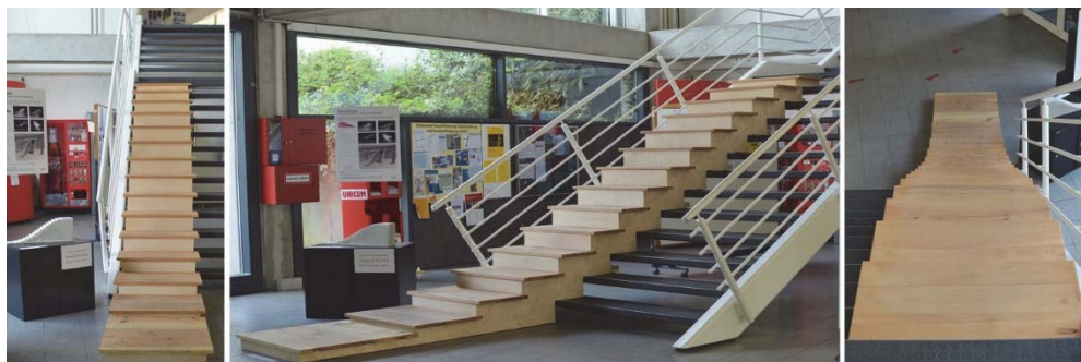
Fig. 7. Installation of the walk-in sinus stairway in the faculty building, 2018. Views from below, from the side and from above
